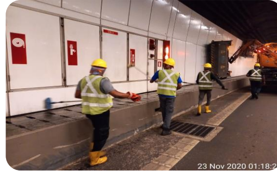
Workers manually cleaning Niches housing sensitive equipment
