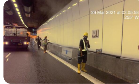
Workers manually cleaning Walkway & Road Kerbs
